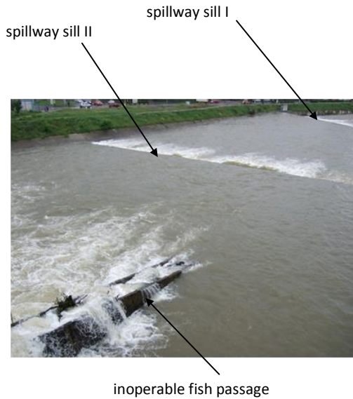
Figure 1 The two spillway sills photo (ABA Someș – Tisa)
